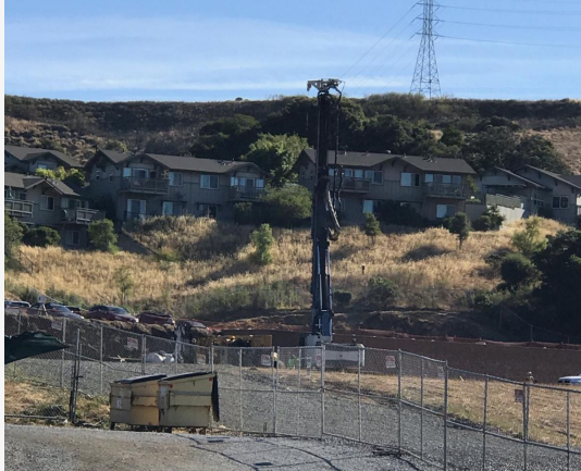
Drill Rig installing piers for shoring walls at Larkspur Landing
