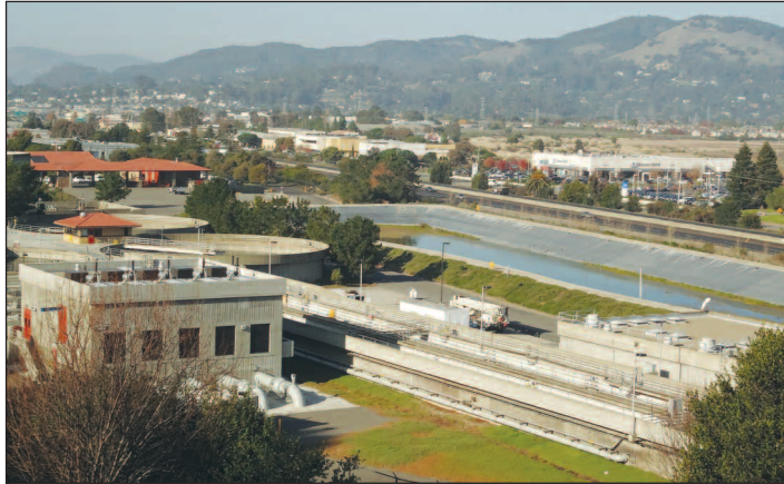
The treatment plant on Anderson Drive near Orchard Supply, serves Ross Valley, San Rafael and Corte Madera customers.
