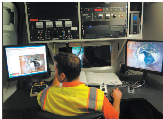
The new CCTV system records images of damaged pipes and pinpoints their exact locations.
