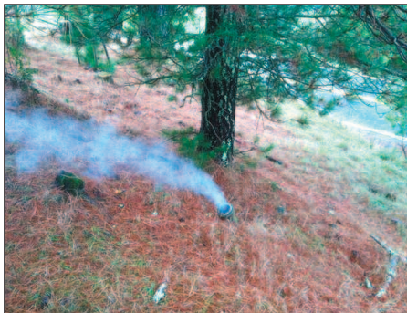
Smoke billows from an uncapped cleanout pipe during the pilot test.
