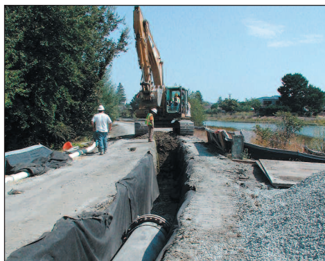
Contractor Maggiora & Ghilotti "turned the corner" on the project in mid-September.
