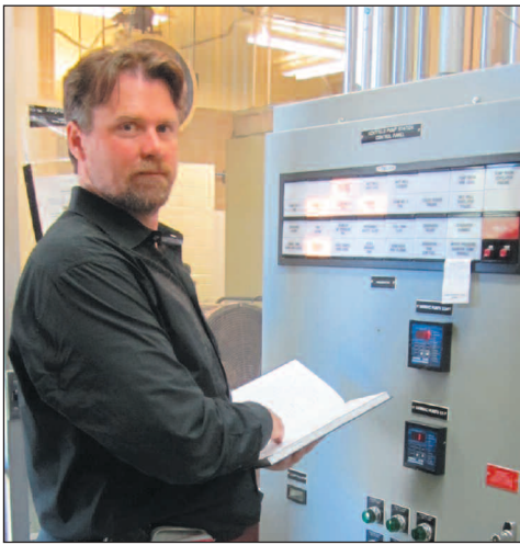
Clark reviews detailed reporting on system performance at Pump Station 15.
